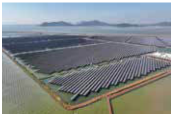
▶ Fishing & PV complementary power Station Municipal investment Group, Guangdong, China
