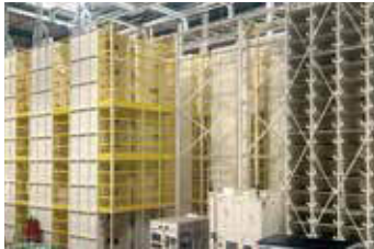
▶ D-BUS energy saving solutions Battery manufacturer, France
