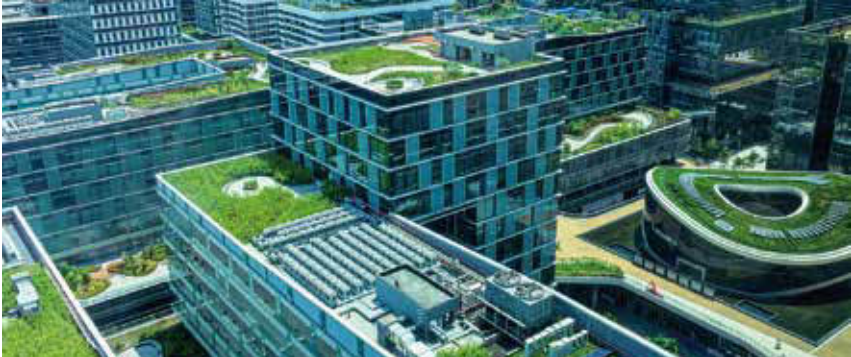
Micro-Grid Energy-Saving D-Bus Solution
