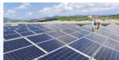
Renewable Power Station
